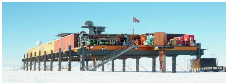
Picture 5.8: Container buildings on the platform scaffolding (Halley V station) (British Antarctic Survey)
