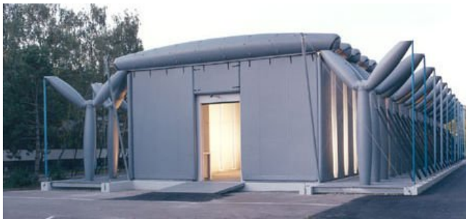
Picture 6.14: Inflatable multi-air-bag cover (type II) (Tarczewski)
