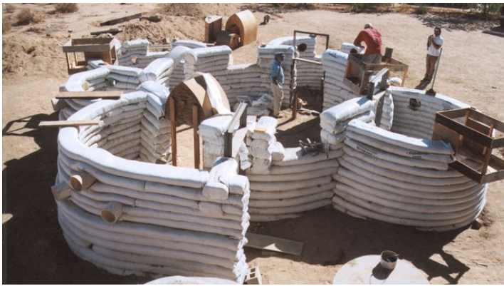
Picture 6.55: Super Adobe construction during building (Cal-Earth)
