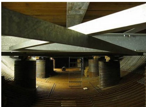
Picture 5.12: The scaffolding for residential containers inside the under-ice tube at the Neumayer station (Alfred Weneger Institute)
