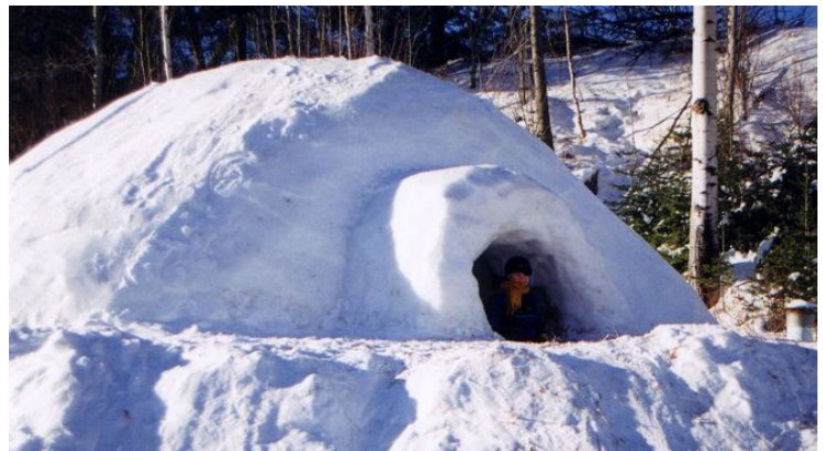
Picture 6.61: Carved out construction in a block of snow
