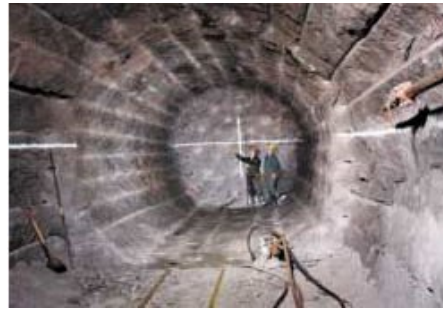
Picture 6.34: The inside of a mining excavation with smooth walls, the underground laboratories in Winnipeg (Kuczyk 2002)
