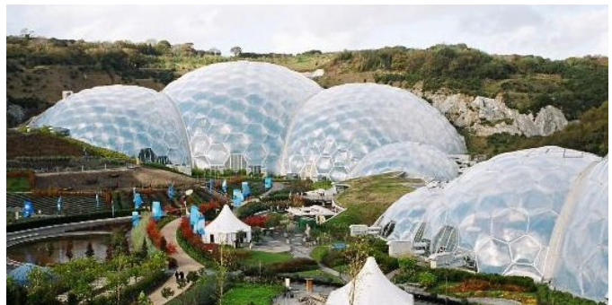
Picture 6.17: Eden Project: metal construction with inflatable panels (Eden Project Ltd.)
