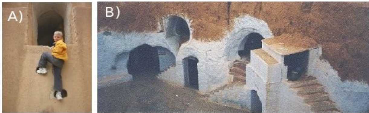
Picture 5.43: Entrance to the second floor is possible with the foot-holes cut out in rock (A) or stairs carved out in rock (B) (Matmata, Tunis)
