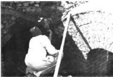
Picture 6.51: The stages of building slanted barrel arch (Petrov 2004)
