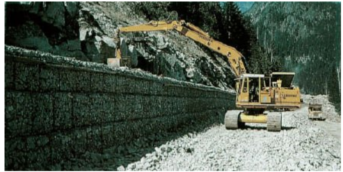
Picture 6.42: Excavator loading gabions (BMTG)
